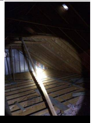
Garage Attic Access
