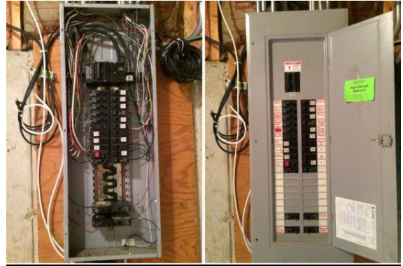
Electric Panel: Improper Screws Used
